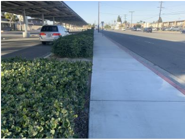
n°. 3 – Sidewalk with no separation in front of Westminster High School on Goldenwest Street (Westminster, California)
