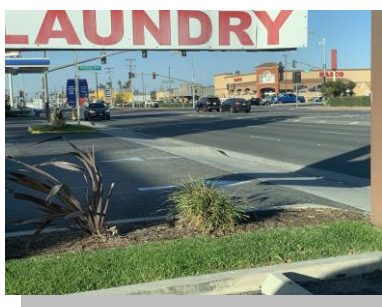
n°. 10 – Four driveway aprons obstruct the sidewalk on Goldenwest Street (Westminster, California)
