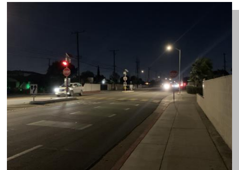
n°. 14 – The flashing red beacon alerts drivers to stop at the intersection. (Trask Avenue, Westminster, California)
